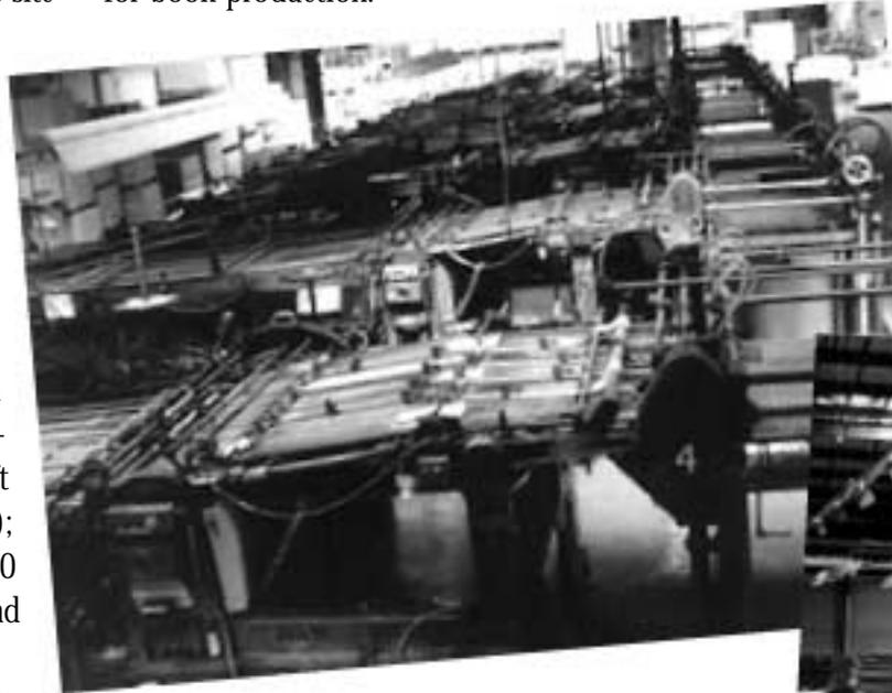
*The picture above shows part of the main machine room and a line of Miehle printing presses. It features seven of these presses, they could print a sheet 52 x 38 inches and had a maximum speed of 2,500 copies per hour.*
